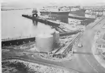
THE NEW tetraethyl lead system of storage tanks and lines is unique at Lago. Ethyl Corporation owns the compound until it reaches weigh tanks in the blending plant.
